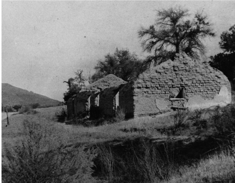
Reed's adobe house c. 1890 after being destroyed by fire. Source: Mill Valley Public Library, Lucretia Little History Room
